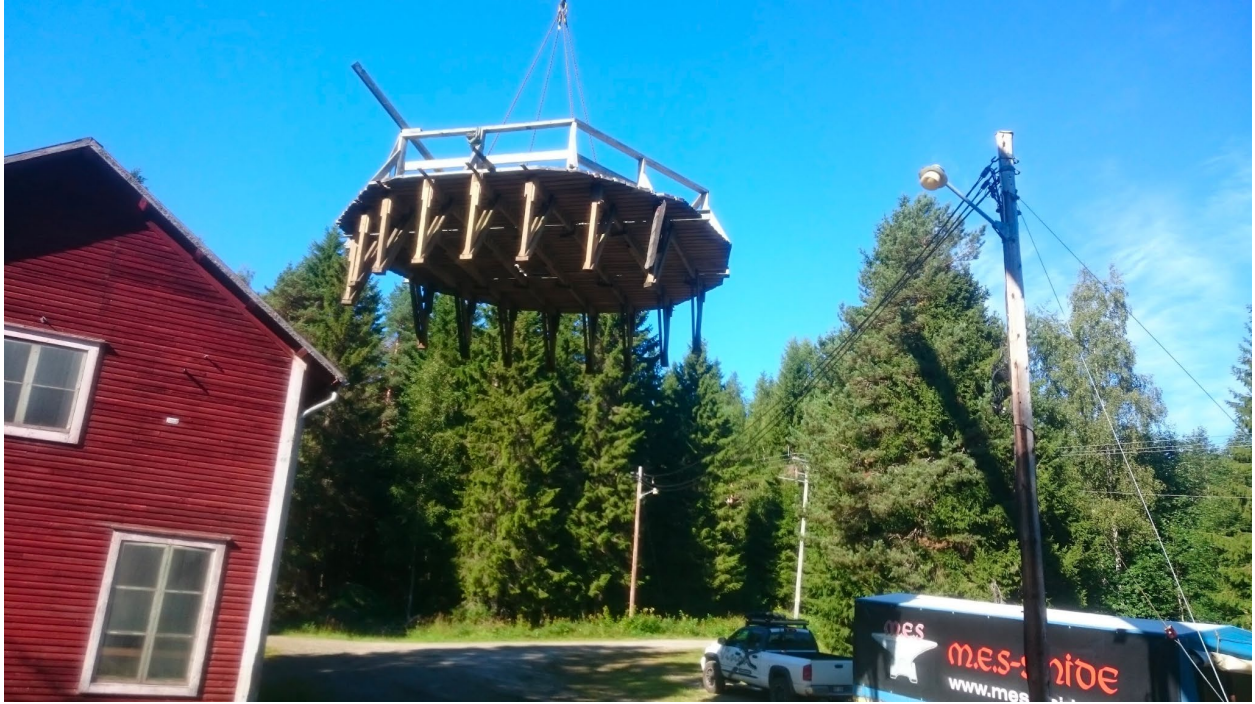
Torntaket lyfts ner.
